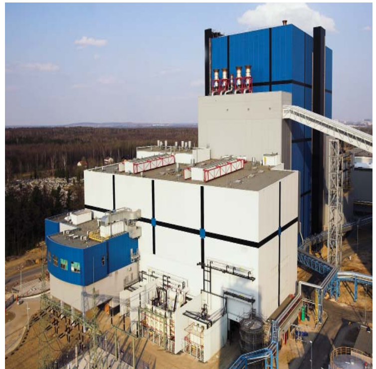
Commercial Operation Begins at the Lagisza Power Plant 460 MWe Supercritical OTU CFB Boiler
