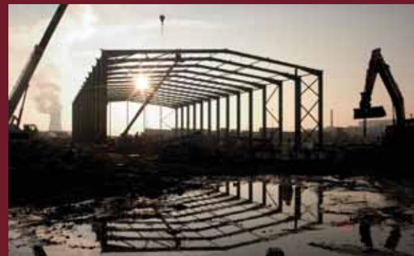
Lay-down area and boiler pre-assembly.
