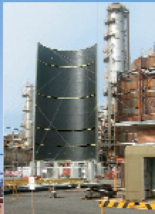
First two radiant panels in place.
