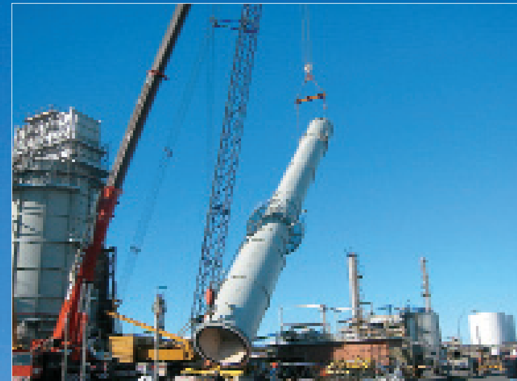
Stack being lifted onto the convection section.
